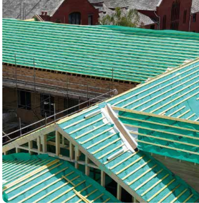
Taiyabah Masjid Mosque, Bolton—Bradley Ascroft Roofing Ltd
