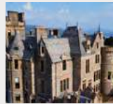
Auchendennan House— DM Roofing & Roughcasting Ltd
