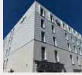
The Marcus Hotel- Thornton Roofing (Ireland) Ltd
