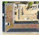
Rushers Ghyll— Clarke Roofing Southern Ltd
