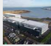
Belfast Harbour Film Studios- Thornton Roofing (Ireland) Ltd
