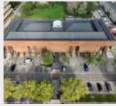
Milton Keynes Library- Ashe Roofing Ltd
