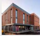
Warwick Hospital- Marksman Roofing & Cladding Ltd
