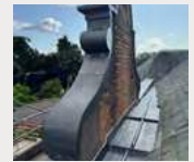
Country Manor— Emerton Roofing (Western) Ltd
