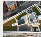
Kellstone— JPT Roofing Ltd, working with Soprema UK
