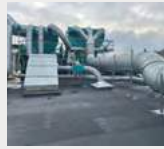
Smurfit Westrock- LRL Roofing Solutions
