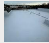
Premier Inn, Margate- Invictus Roofing Ltd
