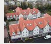
New Road Court Apartments- M. Camilleri & Sons Roofing Ltd
