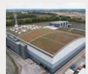
Rivenhall IWMF— MAC Roofing & Contracting Ltd
