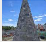
Ellesmere College Turret- Emerton Roofing (Western) Ltd
