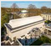
The Library, Murray Edwards College—Millane Contract Services Ltd, working with WestWood Liquid Technologies Ltd
