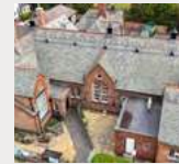
Hoole Community Centre— Emerton Roofing (Western) Ltd
