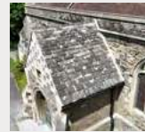
All Saints C of E Church— Richard Soan Roofing Services
