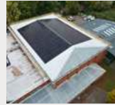
St Nicholas Leisure Centre- Stage Roofing Ltd
