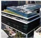
1 Southwark Bridge— Hambro Roofing Ltd
