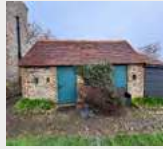
Wickham Manor outhouse- Karl Terry Roofing Contractors Ltd
