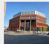
University of Derby Business School— Advanced Roofing Ltd
