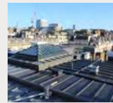
Warwick House— EWN Leadwork Specialists Ltd
