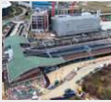
Cambridge South Station- Hambro Roofing Ltd
