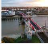
Ferry Footbridge Control Tower- Richard Soan Roofing Services
