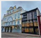
Jersey Opera House—Rateavon (Jersey) Ltd, working with Triflex (UK) Ltd
