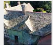
Staick House— Rowlands Roofing
