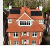
Baslow Road- Clarke Roofing Southern Ltd, working with Keymer Tiles Ltd
