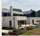
Little Eversden, Cambridgeshire- Roof Brothers Ltd, working with CUPA PIZARRAS S.A.
