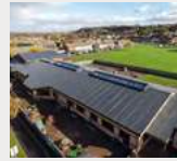
Nant Caerau Primary School- J Randall Roofing Contractors Ltd
