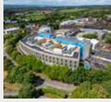
Countess of Chester Hospital- Longworth Facades
