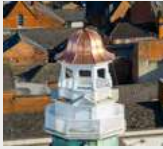
The Highcross Bell Tower- Prestige Metal Roofing Ltd
