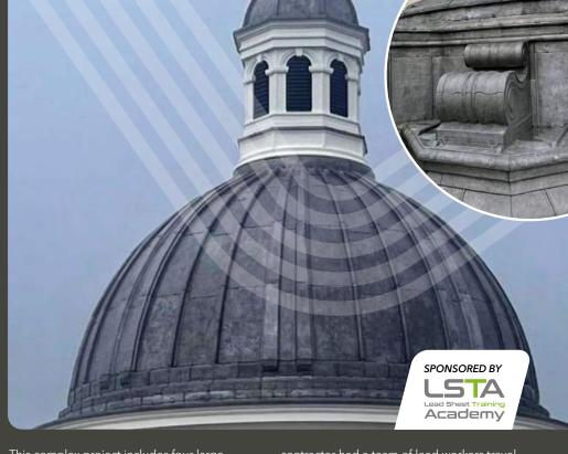
This complex project includes four large scrolls. The lower parts were shaped to match the original timber pattern, while the top scrolls featured original spun timber encapsulated in lead. This London-based
