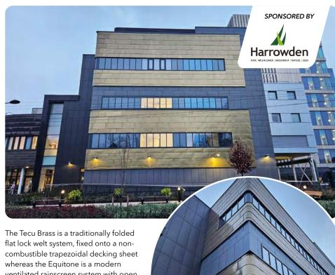
ventilated rainscreen system with open gap joints between the panels fixed back to a non-combustible composite panel.
