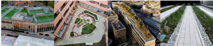
Eclipse Leisure Centre— D F Roofing Ltd
