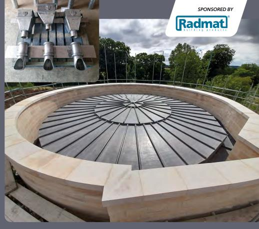
The site had fallen into disrepair over the years and had been placed on Historic England's Heritage at Risk Register. The leadwork on the tower was completed in three phases, the first being the gutters, which were no more than 400 mm wide and deep sided, with the lowest point being around 1.3 m below the main roof, and with an abutment on the outer edge with some of the code 8 rolls weighing
